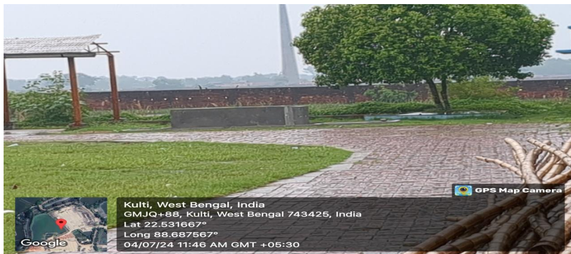
Solid Waste Management Facility
